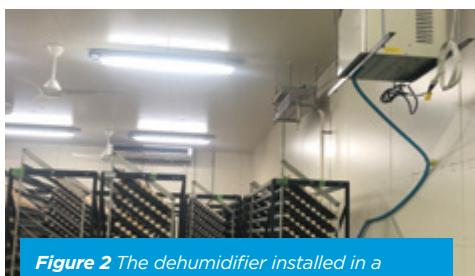
**Figure 2** The dehumidifier installed in a higher position which gives enough distance from the eggs in the egg store.
