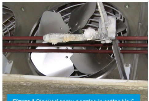
Figure 1 Blocked spray nozzles in setter No.6
